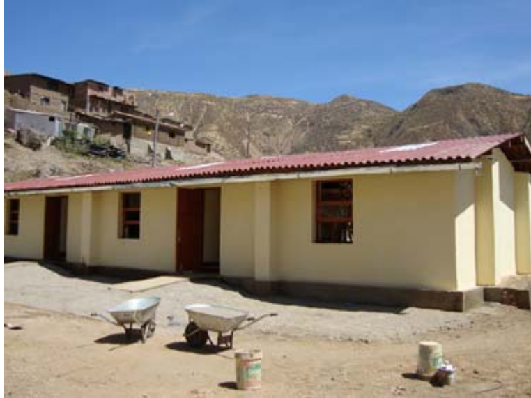
The finished school is safer and more attractive. Courtesy of GHI/Stanford/PUCP
