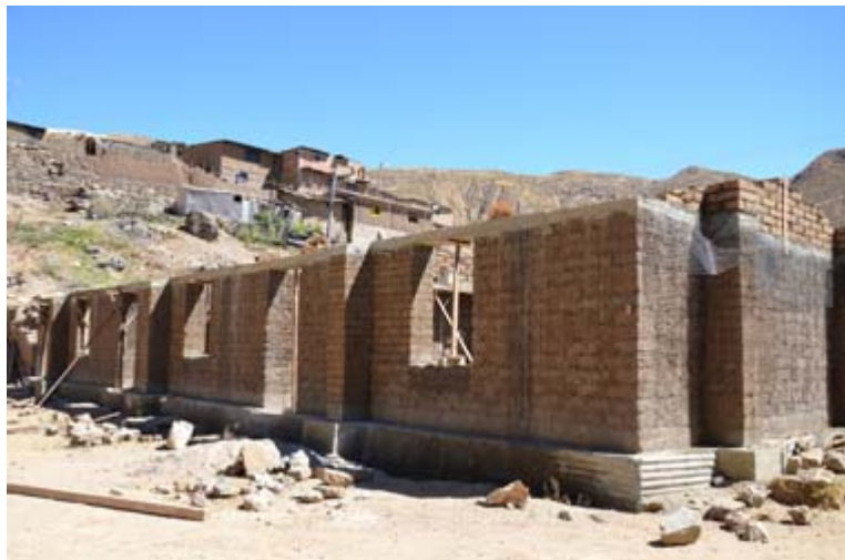
Geomesh is applied to both the interior and exterior walls. Courtesy of GHI/Stanford/PUCP
